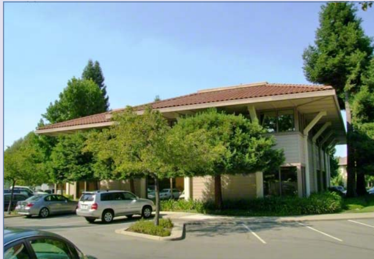
3240 W. Stone Valley Road Alamo
